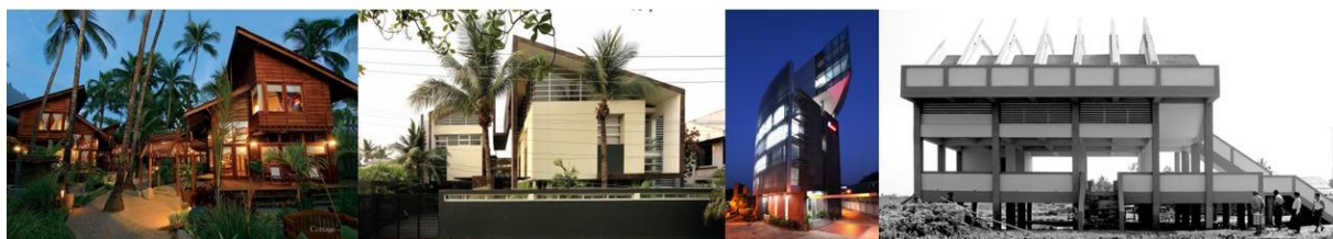
Figure 2. (Left) Amata Resorts & Spa, (Center Left) MG Residence, (Center Right) MDG Headquarters, (Right) Cyclone Shelter (Source: Spine Architects).
