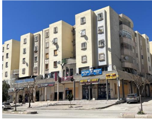
Figure 4. Mixed-use in Mid-rise apartments.
