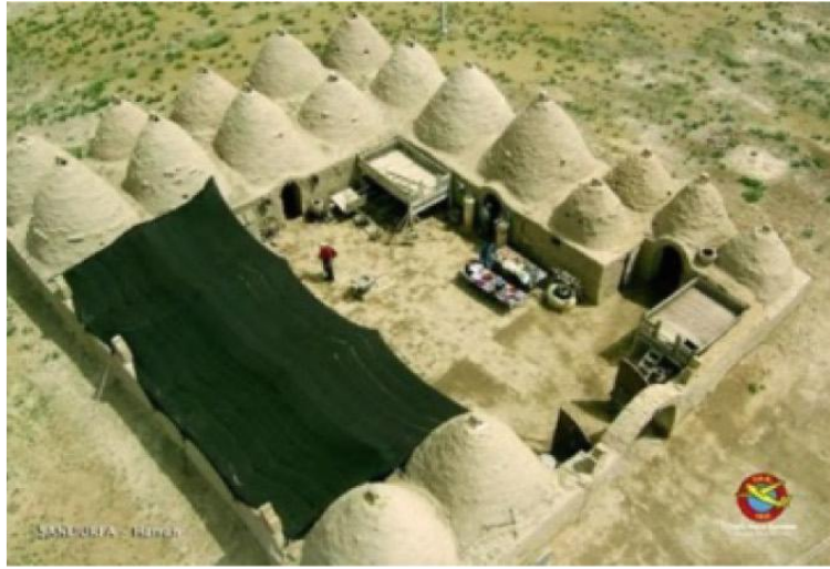
Figure 2. Courtyard plan form (a) and aerial views of the Harran conical domed houses (Sanliurfa Regional Council for the Conservation Cultural Heritage of Ministry of Culture and Tourism Archive, 2026).
