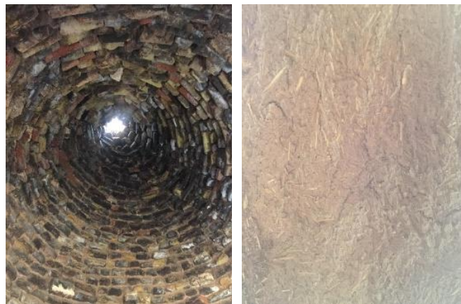
Figure 3. Corbelled Conical Dome Structure and Wall of Harran Domed Houses (Akalp, 2025).
