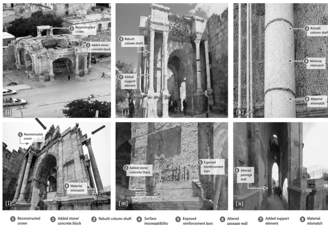
Figure 5. Inappropriate restoration of the Gate of Caracalla: (i) general view of the monument; (j) frontal view showing reconstructed columns; (k) detail of column reconstruction using incompatible materials; (l) lateral view of the arch highlighting structural imbalance; (m) use of reinforced concrete and exposed metal bars; (n) interior passage showing alterations to the original structure. (Source: Author, 2026).
