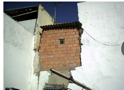
Figure 1. Construction of an unfinished room in red brick on a terrace. Photo A. Boutemedjet, 2022.
