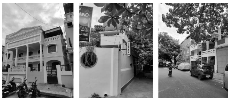
Figure 5. Puducherry: details of coloured edges (site inspection, 2025).
