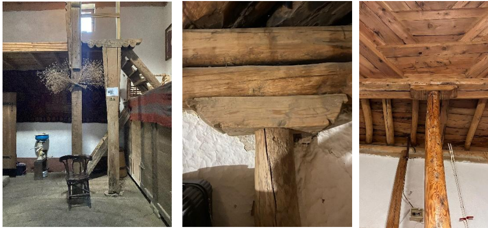
Figure 4. Structural and symbolic elements of the kirman ceiling system: the gelin direği (bride’s post), the post capital, and the main post, respectively from left to right (Personal Archive of Seval Akbulut, 2026).
