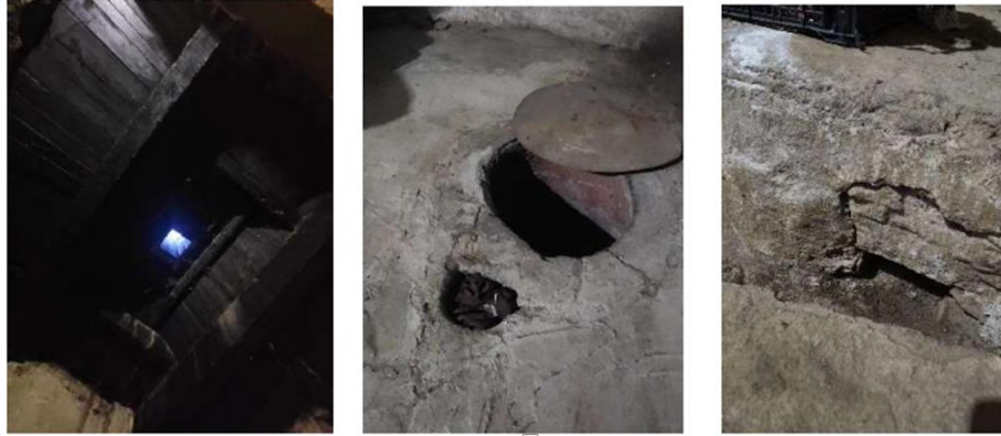
Figure 1. Components of the tandır system in traditional Bayburt houses: the chimney above the tandır, the tandır with its ventilation system, and the tandır ventilation system, respectively from left to right. (Personal Archive of Seval Akbulut, 2026).
